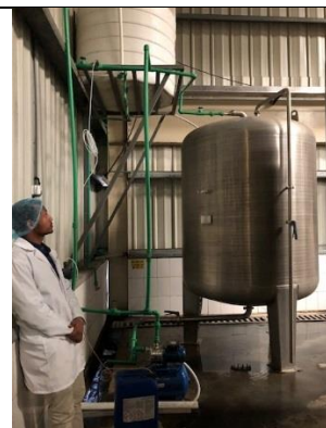
First Filtration: Sand Filter
