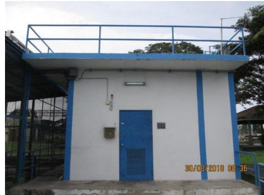
Deep well house (old style)
