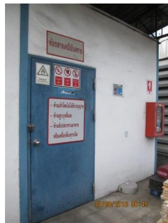
Chemical storage room
