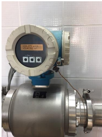
Water Flow Meter Installed in Deep Well House
