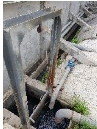
Wastewater discharge point
