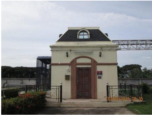
Deep well house (new style)
