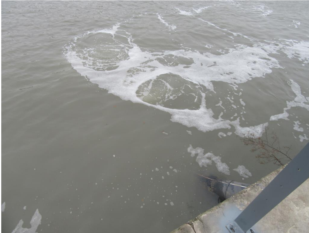
Wastewater finally discharge point
