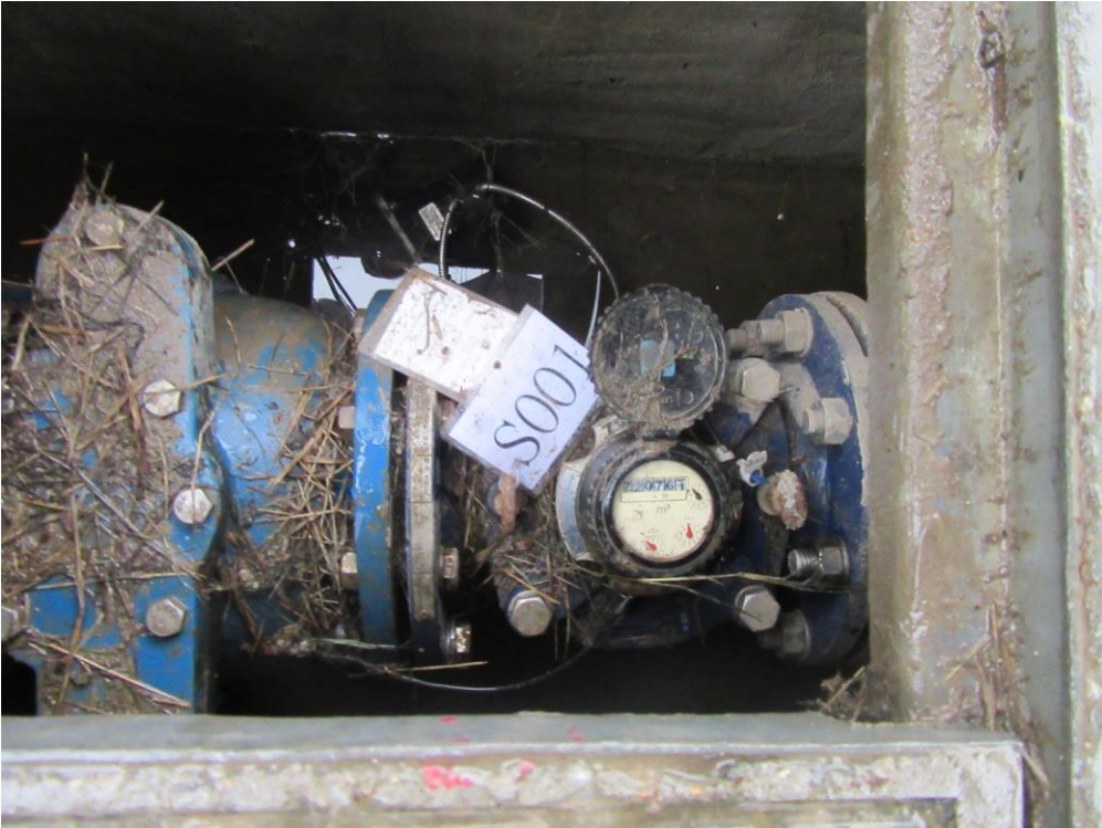
The water flow meter
