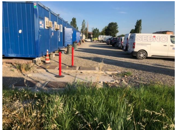
Outlet water (point of discharge)
