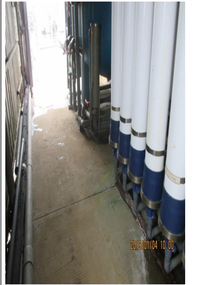
Before: The coffer was damaged in the wastewater treatment plant. Next was a small river.
