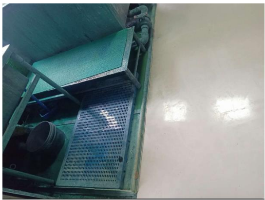
After: The pipeline is repaired, and remodify the room. The tray is used as secondary container.
