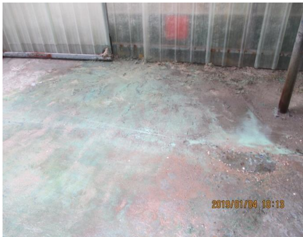
Before: Some leaking on the ground.
