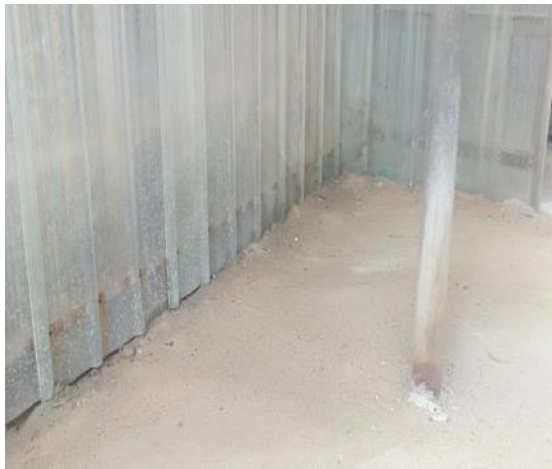
After: The leaking is clear.
