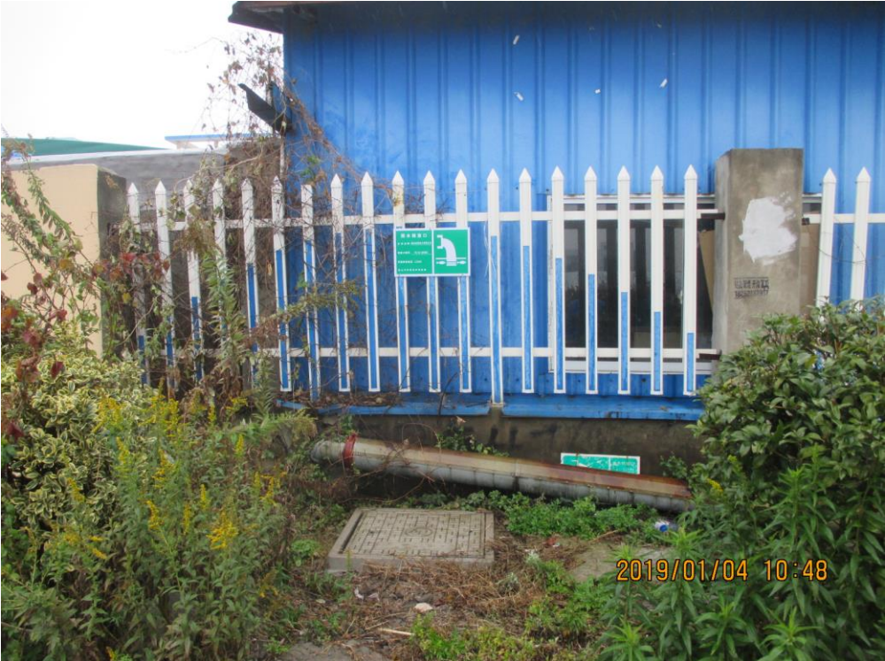
Rainwater discharge point
