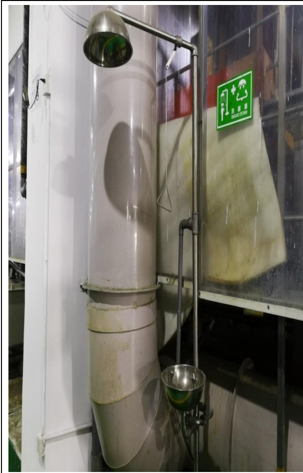
Before: The washing water of one eyewash would be discharged to the ground.
