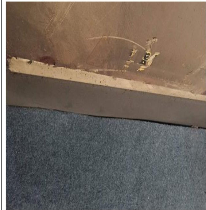
After: The oil absorbent felt is equipped.
