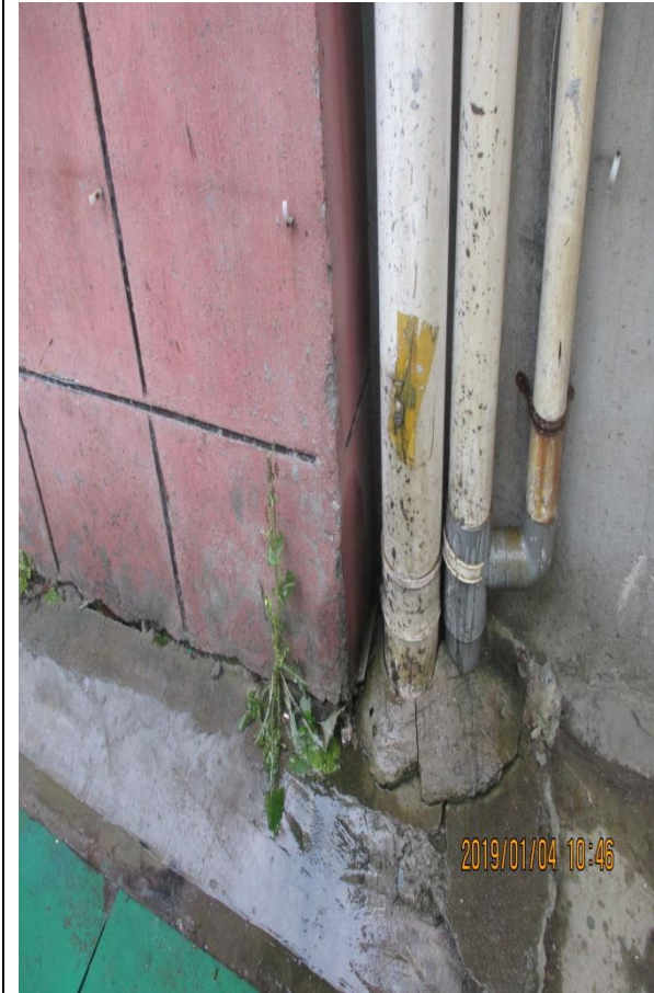
Before: Roof rainwater pipeline was broken.
