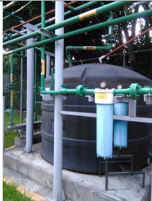
Waste water Tanks for irrigation from Residual water treatment plant
