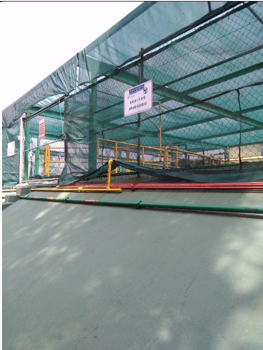
Residual water treatment plant
