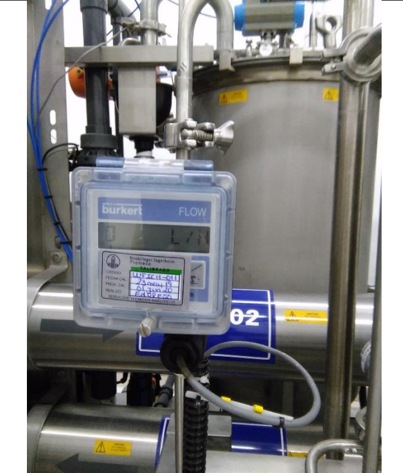
Industrial water treatment plant
