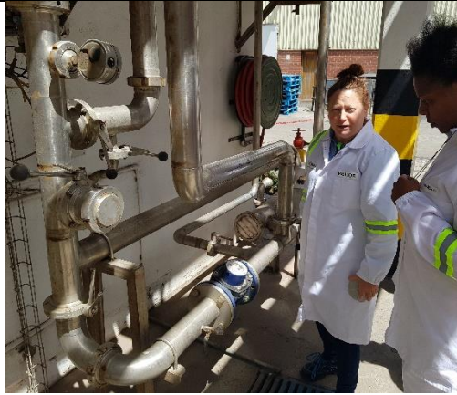
Water Flow Meter
