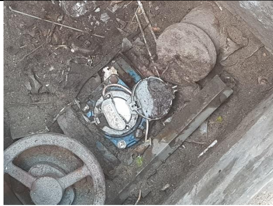
Incoming Water Meter
