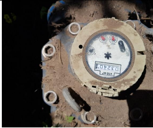
Incoming Water Meter
