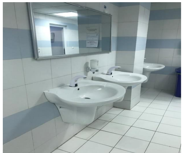
Sensor operated faucets installed at employee's canteen
