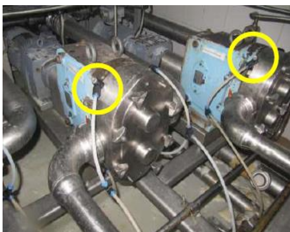
Flow Controllers installed to reduce water consumption
