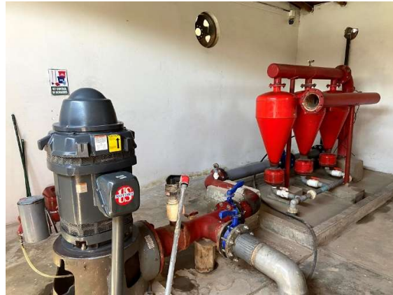
Raw water collection and pumping system
