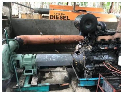
Irrigation Catchment Pumping System
