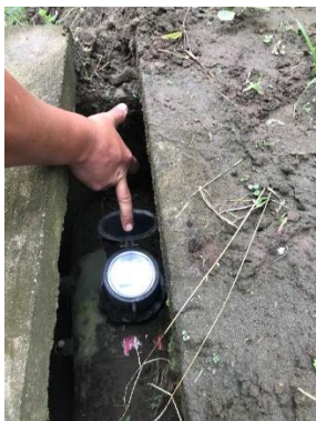
Surface Water Flow Meter for Irrigation
