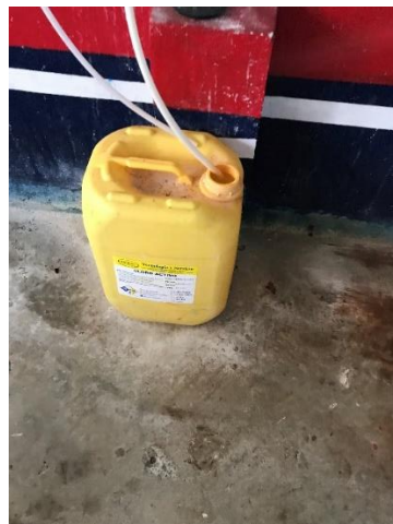
Chemical Application for Recirculating Water
