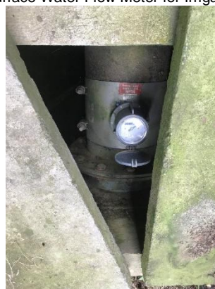
Surface Water Flow Meter for Irrigation
