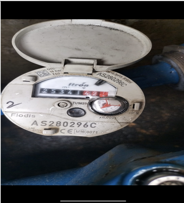
Main Water Flow Meter
