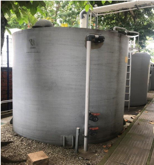
Rain Water Storage Tank at BAT Singapore
