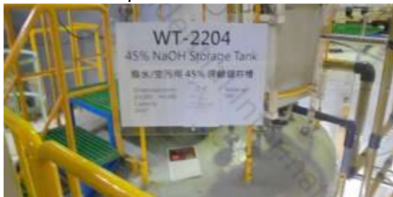
Wastewater NaOH storage tank
