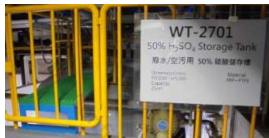
Wastewater H 2 SO 4 storage tank
