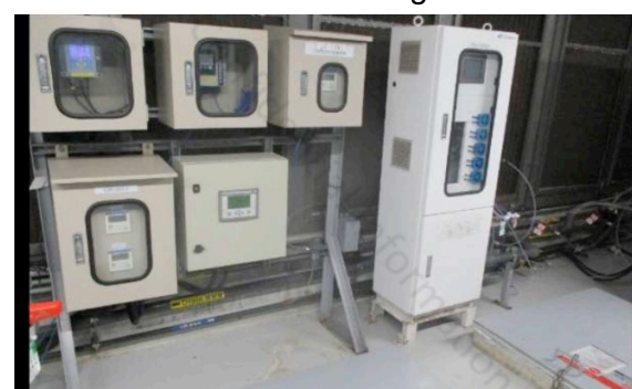
Effluent Water Quality Monitor Instrument
