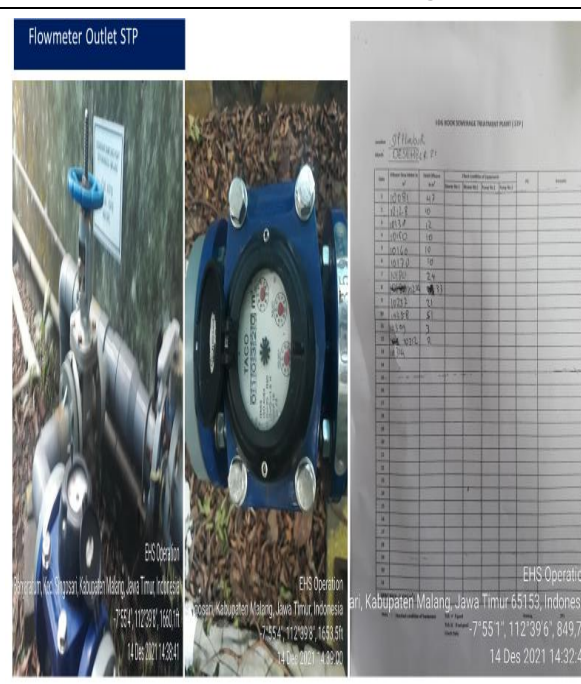
STP Outlet Flow Meter &amp; Log Sheet
