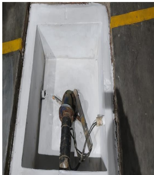
Submersible Water Pump
