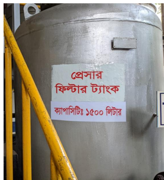
Pressure Filter Tank ETP
