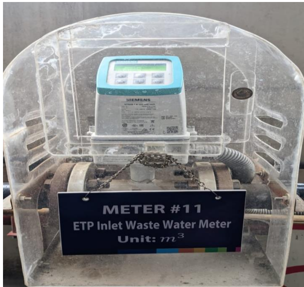
ETP Inlet Flow Meter
