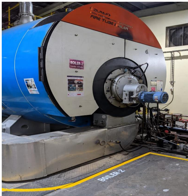
Boiler 12 Ton/hr
