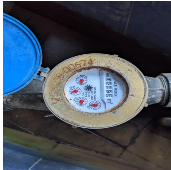
ETP Outlet Flow Meter
