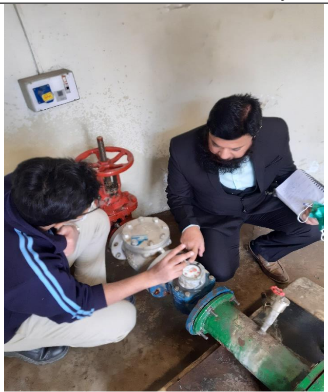
Inspection of Tube well # 2 Flow meter
