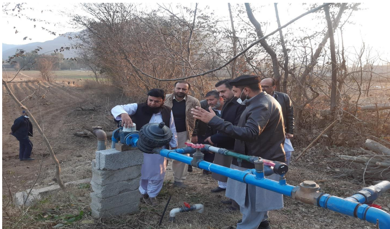
Drip Irrigation Flow Meter at site Catchment
