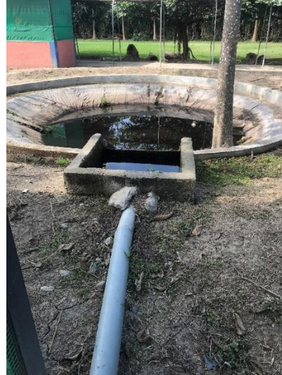
Process Water Treatment System - Solids Decantation prior to discharge.
