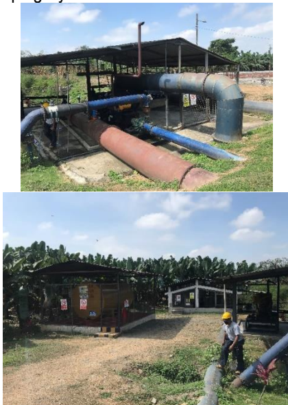
Pumping System for Process Water Discharge
