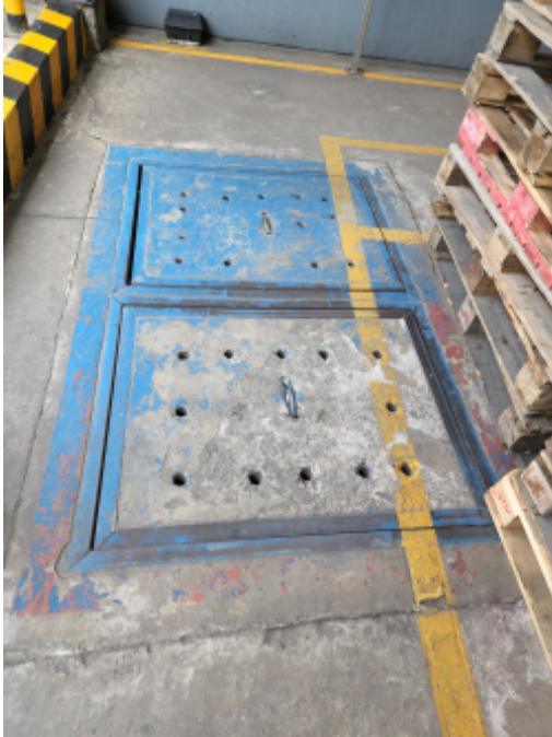
Storm water drain on site.jpg
