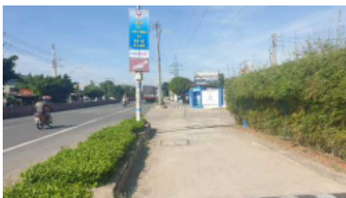
Street view of the La Vie Tan An water bottling plant.jpg
