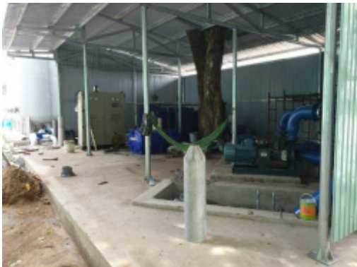
LAWACO new water treatment system.jpg
