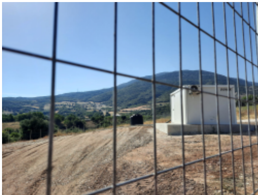
New well not connected to site yet.jpg
