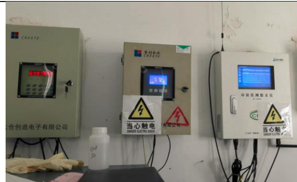
Photo 5: Online monitoring devices installed for treated effluent
