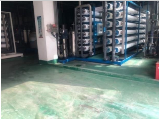
Photo 4: Newly installed facility for purifying reclaimed water
