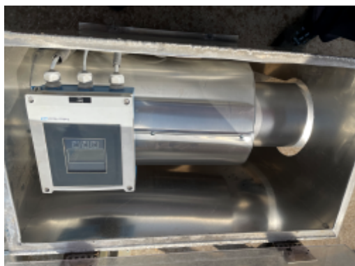
Each well has a meter for recording water withdrawal well meter.jpg
