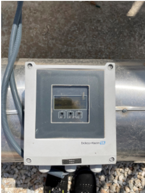
Example of a typical water meter used to monitor withdrawals Water meter.jpg
