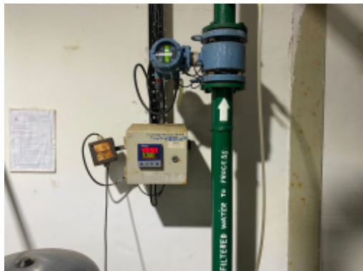
Flowmeter for Filtered water to Process.JPG
