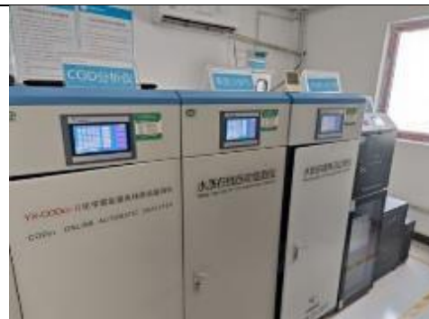
Photo 8: Onling Monitoring Devices Installed for Treated Effluent at Site Wastewater Treatment Station
