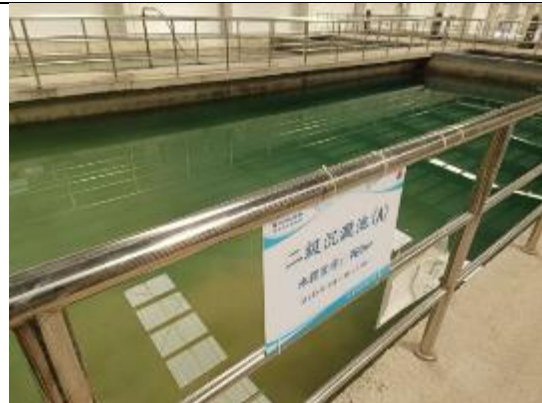
Photo 4: Secondary Sedimentation Tank
