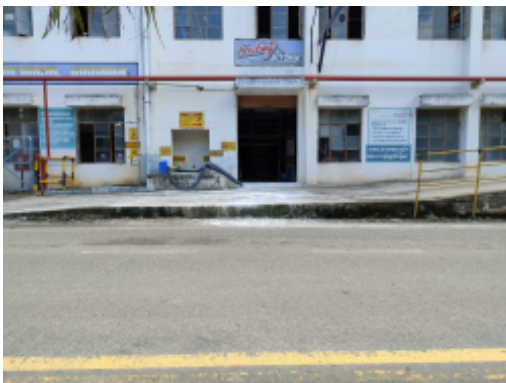
chemical spillage near vaccum pump station.jpg
