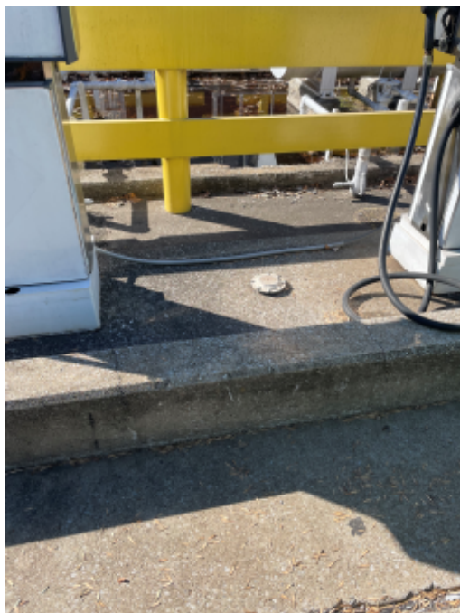
Bunding at fuel storage and dispensing area.jpg
