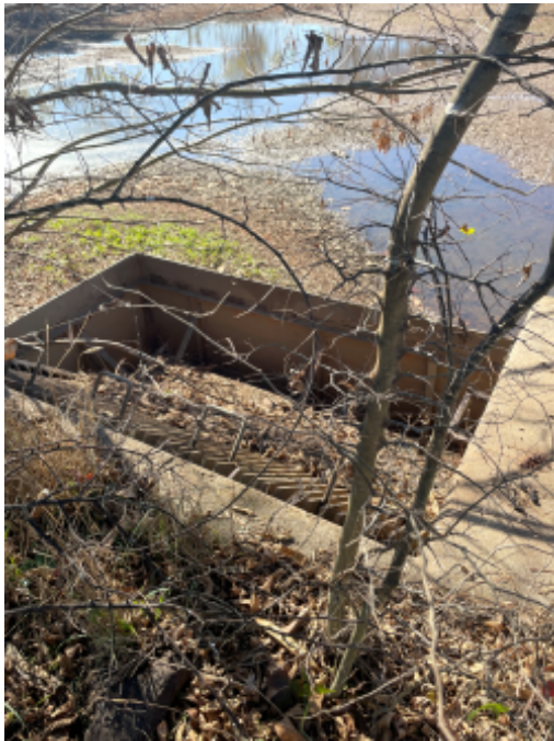
Overflow weir of stormwater detention pond.jpg
