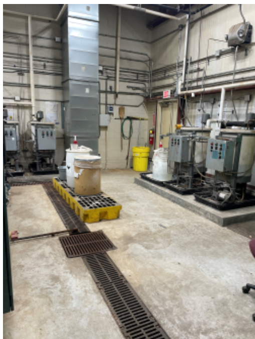
Production chemicals on spill trays.jpg
