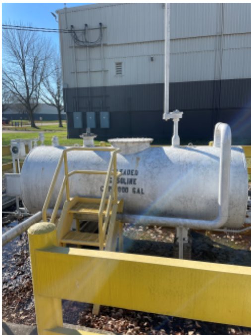
Fuel storage tank with bunding.jpg
