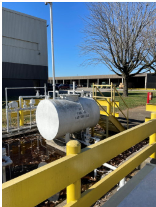
Fuel storage tank with bunding photo 2.jpg
