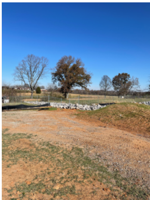
Rock lined (rip) stormwater drainage channel from detention pond under development in new construction area.jpg
