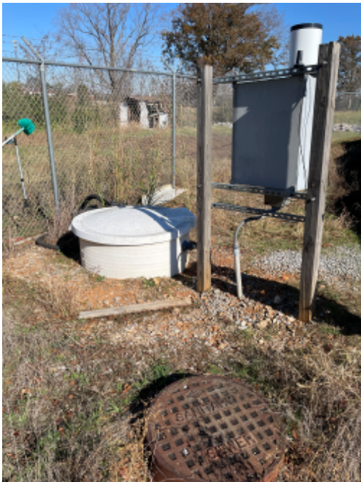
Sanitary sewer maintenance hole where effluent leaving the site is metered for flow.jpg
