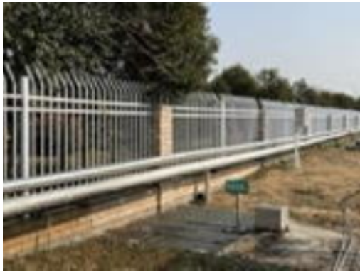
Rain water discharge point.JPG
