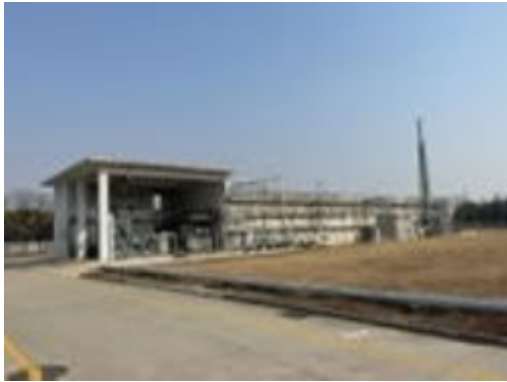
Wastewater treatment plant.JPG
