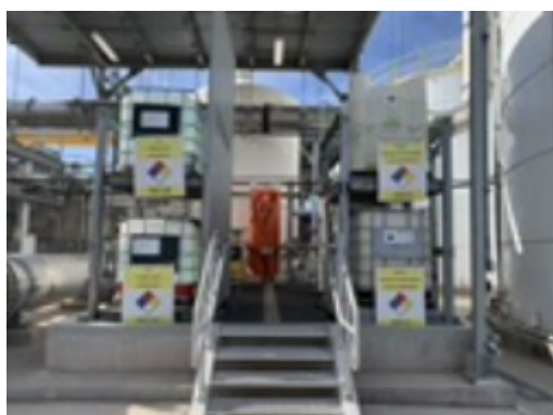
Water Treatment and Reclaim Recovery (WATR) citric acid storage and drench station.jpeg
