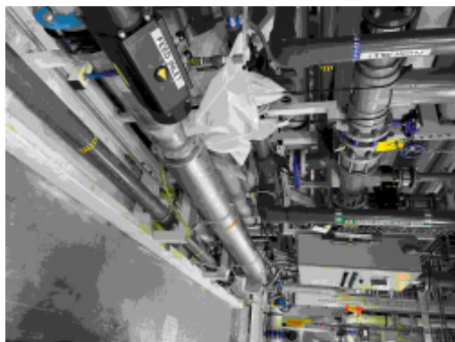
019 Witches hat capturing water leaks in UPW system_00.jpeg
