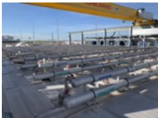
Water Treatment and Reclaim Recovery (WATR) pipework for UFP UF permeate and MPA.jpeg
