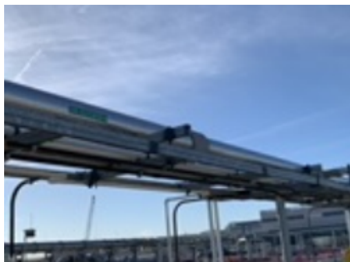
Water Treatment and Reclaim Recovery (WATR) utility water line.jpeg
