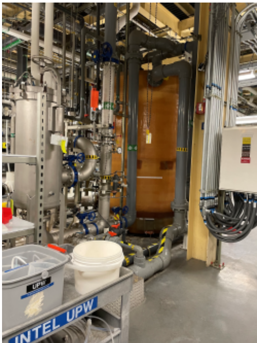
010 RO System Cleaning Tank.jpg
