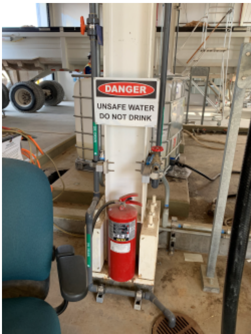
Water Treatment and Reclaim Recovery (WATR) water connection labelling.jpeg
