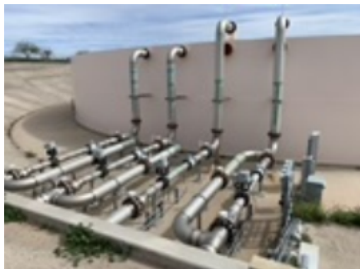
Blended Reclaim Water (BRW) Tank pipework.jpeg
