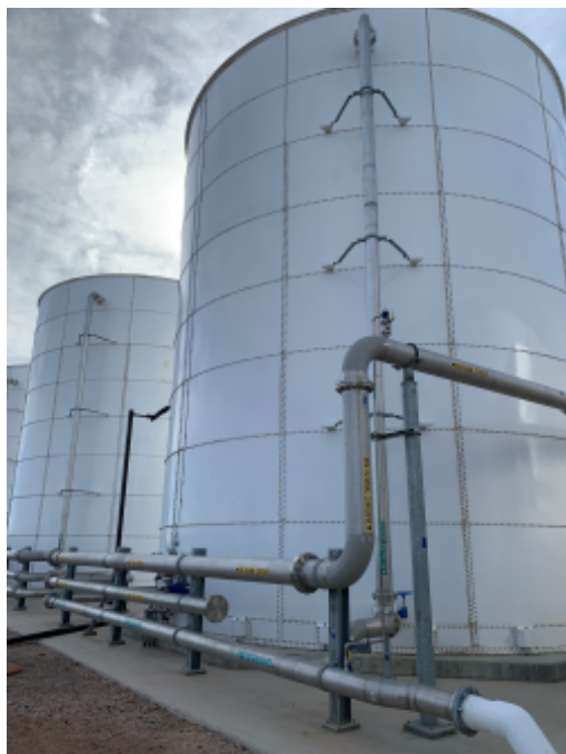
Water Treatment and Reclaim Recovery (WATR) tanks and pipework.jpeg
