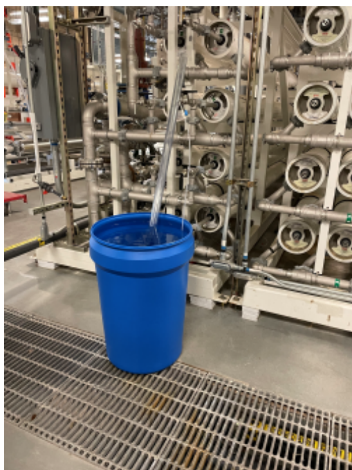
005 RO filter cleaning tank.jpg
