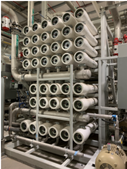
Water Treatment and Reclaim Recovery (WATR) Reverse Osmosis Plant.jpeg
