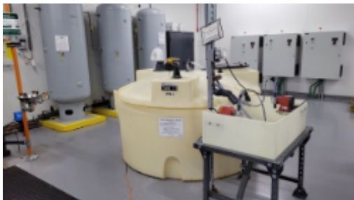
Sodium Hypochlorite storage tank in a chiller room.jpg
