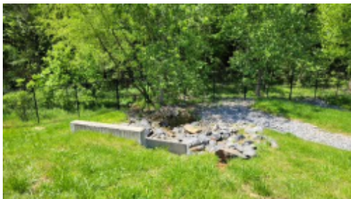
Rip rap downstream of wet (stormwater) pond leading to site boundary and South Fork (Catawba) River.jpg
