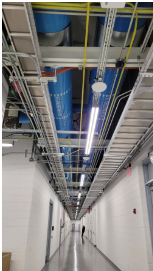
Chilled Water pipework in a data centre hallway.jpg
