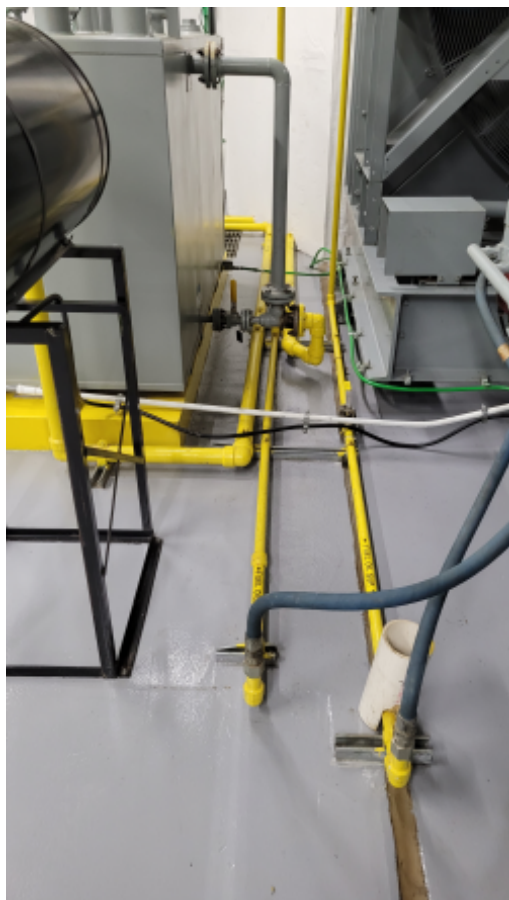
Fuel oil pipes in generator room.jpg
