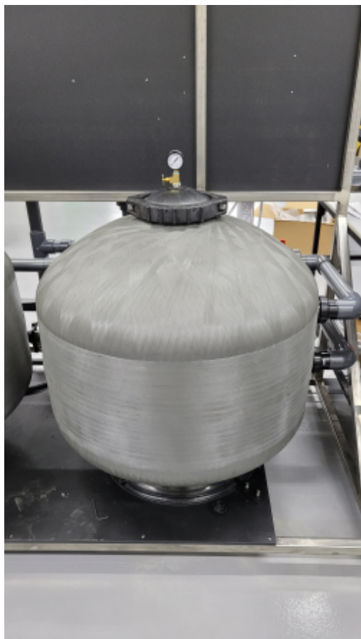
Tank into which ProMoss is placed in a chiller room.jpg
