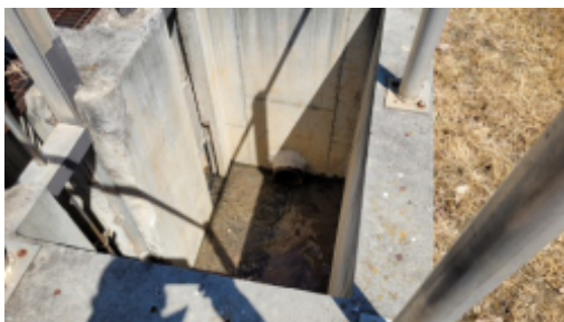
Domestic effluent (sewer) prior to entry into bioretention pond 3.jpg
