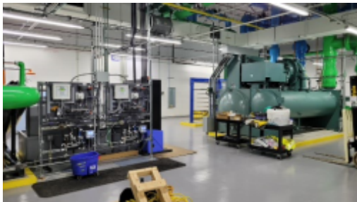
ProMoss water treatment system adjacent to a chiller.jpg
