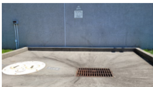
Diesel Underground Storage Tank (UST) with bunding for fuel delivery.jpg
