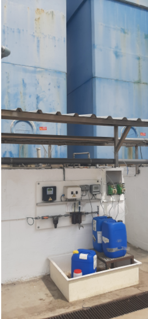
Dosification point, cooling towers.jpg
