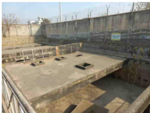
Storm Water Wanks and Infiltration wells.jpg
