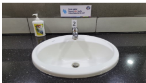
Office restroom basin.jpg
