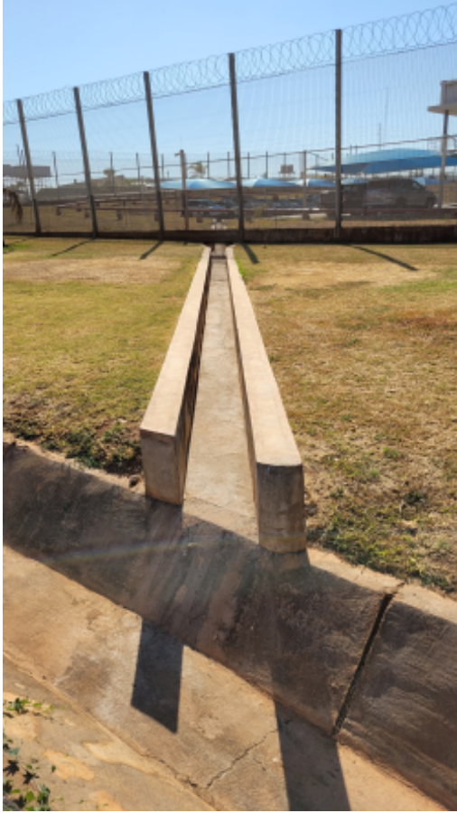
MFEZ stormwater system adjacent to the site 2.jpg
