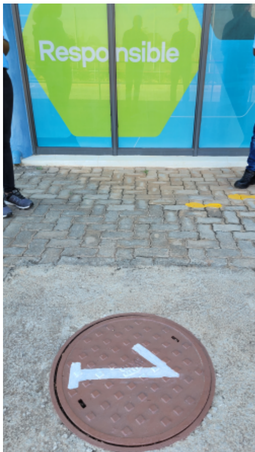
Outside sewer manhole.jpg
