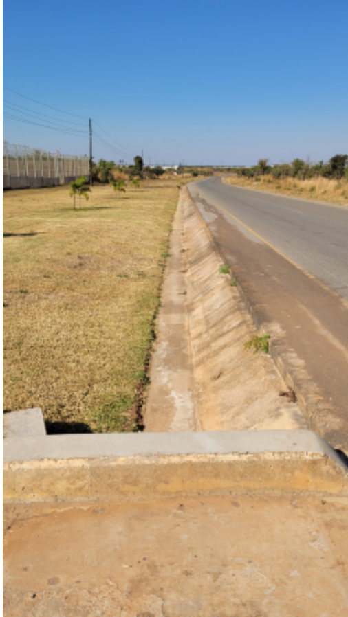
MFEZ stormwater system adjacent to the site 3.jpg
