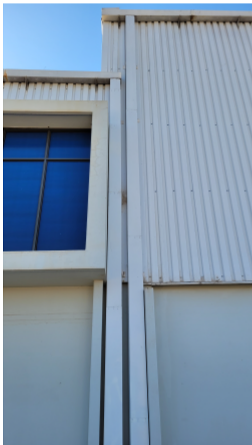
Stormwater system from roof 2.jpg
