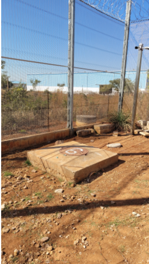
Site effluent egress point into MFEZ effluent pipeline system.jpg
