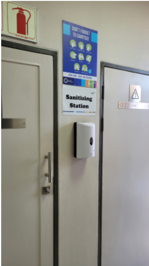
Office sanitation station.jpg
