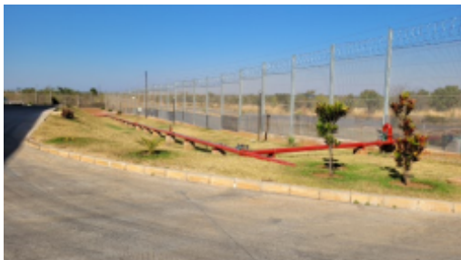
Input water pipeline.jpg
