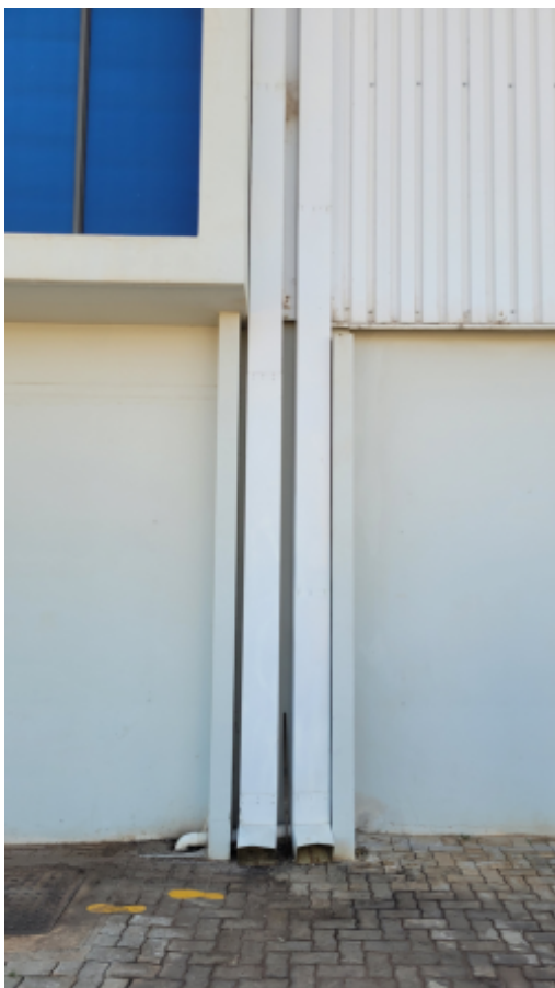
Stormwater system from roof.jpg
