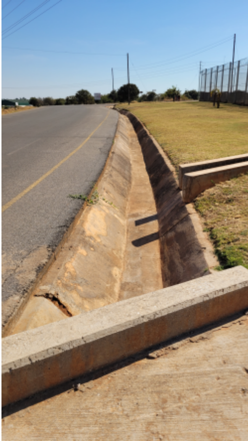
MFEZ stormwater system adjacent to the site.jpg
