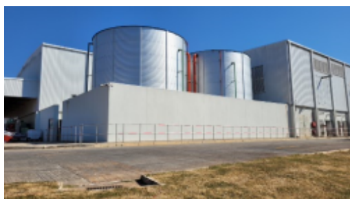
Site water storage tanks.jpg
