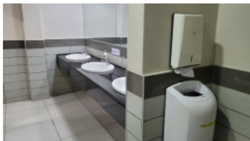
Office restroom basins.jpg
