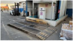
Fuel dispensing area without any spill prevention system other than bunding for the fuel pump.jpg
