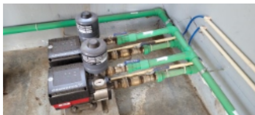
Pumps for the site water storage tanks.jpg
