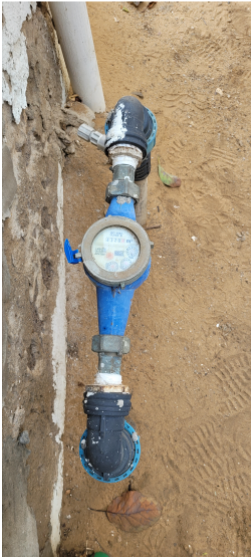
Meter to pumps from above ground water storage tanks.jpg
