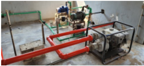
Pumps for the site water storage tanks and fire suppression system.jpg
