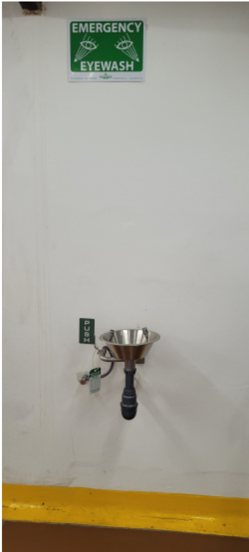
Eyewash station in factory near chemical storage.jpg
