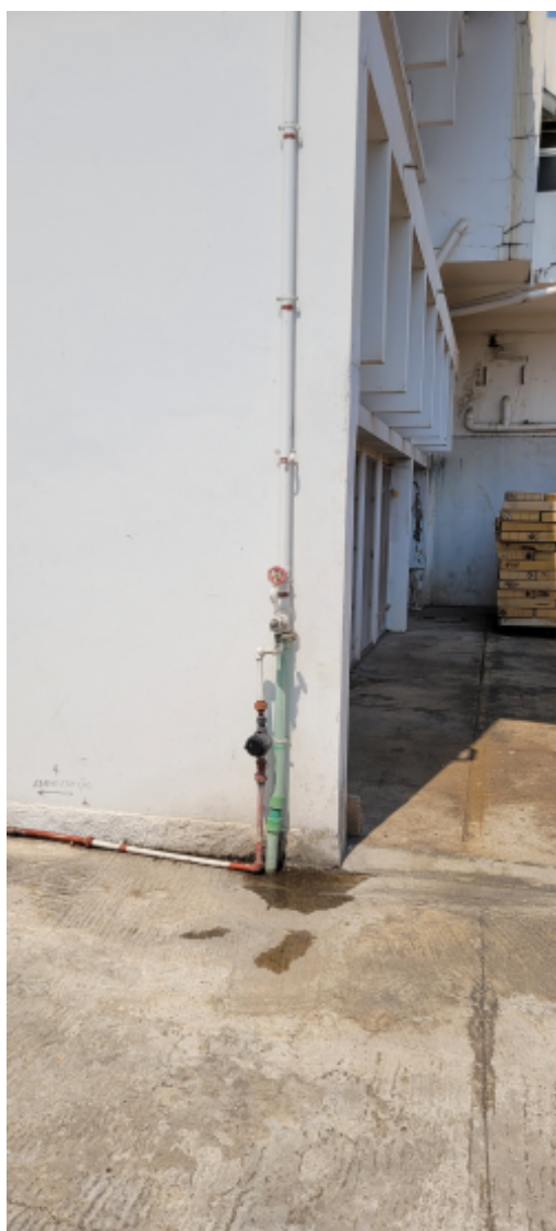
Minor water leak outside of the office building.jpg
