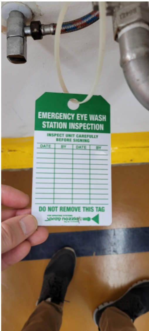
Eyewash station next to factory chemical storage with maintenance card not completed.jpg
