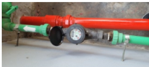
Meter for the site water storage tanks pipework.jpg
