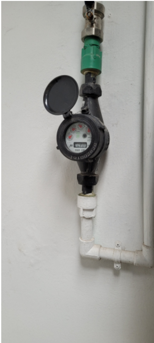
Water meter and pipework inside the factory for the cooling tower.jpg
