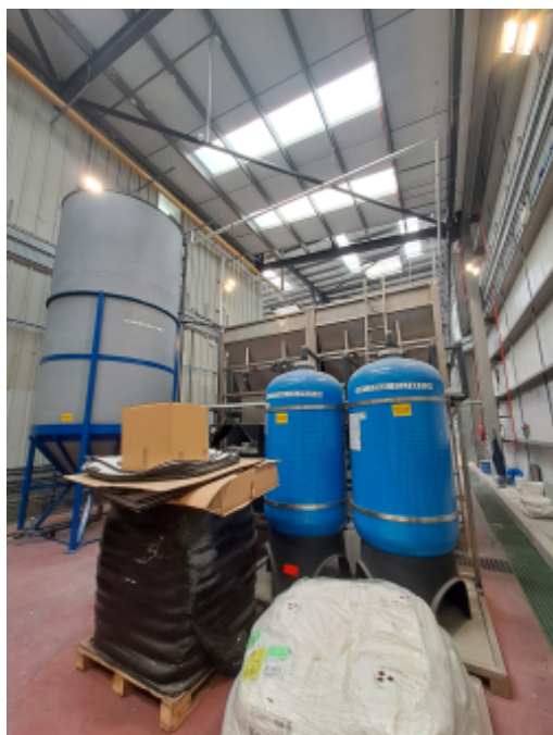
Anodising line WWTP with separate acid treatment line.jpg
