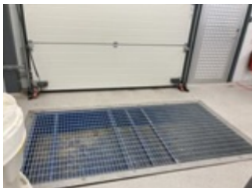
Spill tray in nicotine storage room - not connected to water infrastructure.JPG
