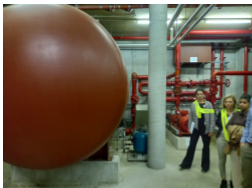
Pressure tank for Sprinklers 2.jpg
