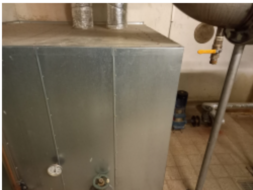
Neutralization tank.jpg
