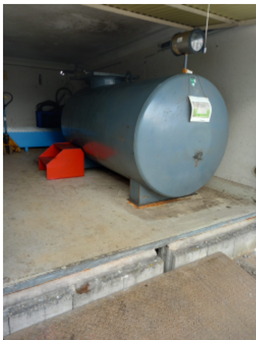
Waste Oil Tank - no spill kit.jpg
