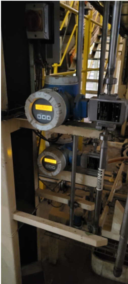
Digital water meters in factory.jpg
