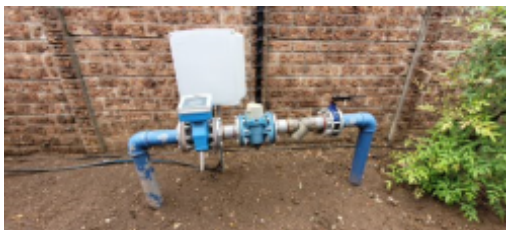
Incoming water line and meter.jpg
