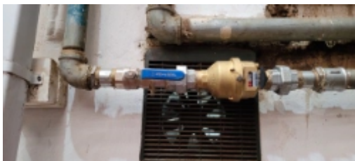
Shut-off valve and meter in factory.jpg
