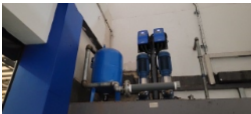
Booster pumps for storage tanks for production.jpg
