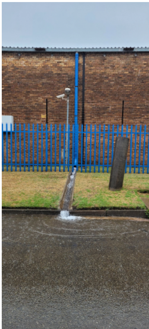
Rainwater flowing off site from the warehouse roof.jpg
