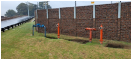
Exterior meter and fire suppression connections.jpg
