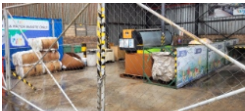
Waste handling area with no bunding or stormwater run-off capture.jpg
