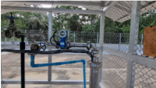
Sealed Metering Shallow Well.jpg
