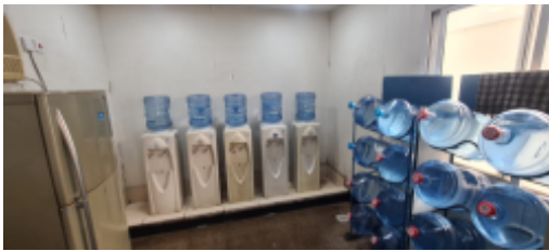
Drinking Water Station.jpeg
