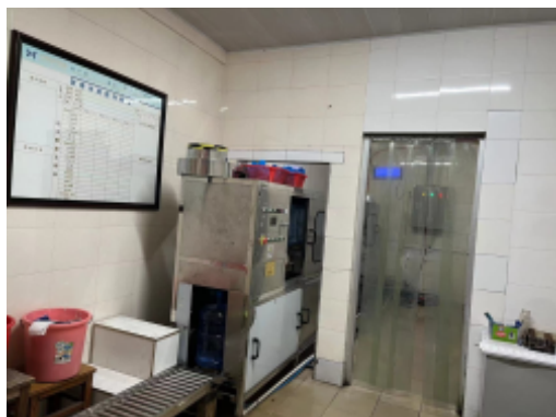
Drinking water filling area-Furong Plant.jpg
