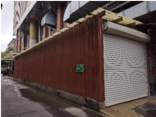
Non-hazardous warehouse-Tuanjie plant.jpg
