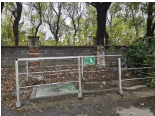
Domestic wastewater discharge point-Tuanjie Plant.jpg
