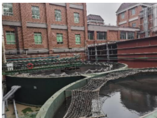
Wastewater treatment-Tuanjie Plant (1).jpg
