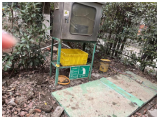
Domestic wastewater discharge point-Furong Plant.jpg
