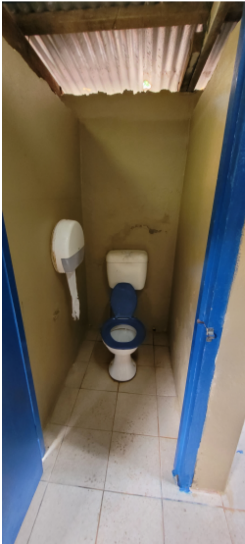
Toilet near Mechanical maintenance area.jpg
