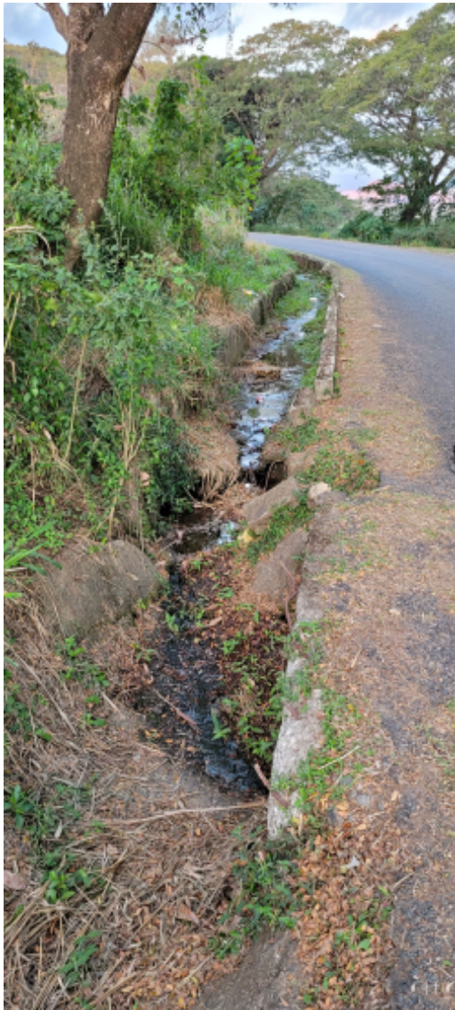
Stormwater drain outside the site on western side.jpg
