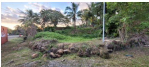
Pond (very likely artificial) within the on-site stormwater system.jpg
