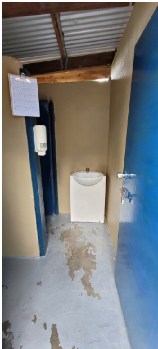
Bathroom near Water Storage Tanks.jpg
