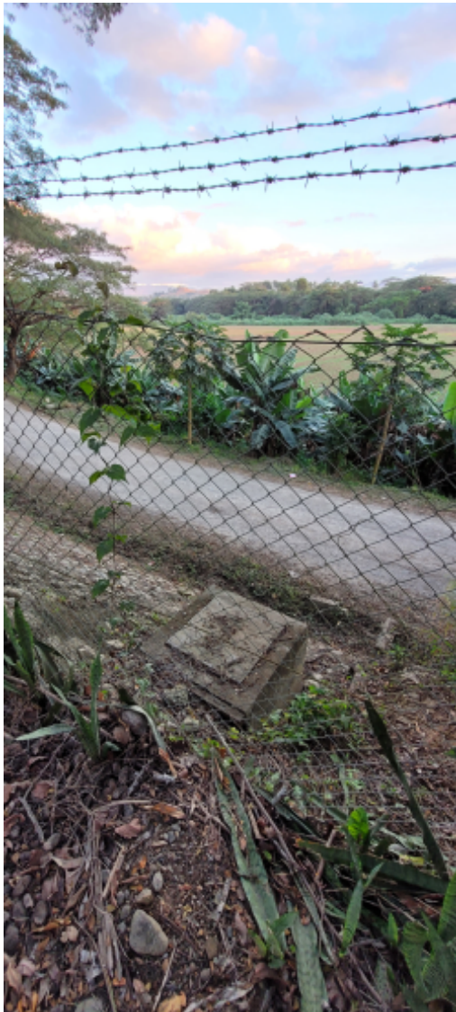
Stormwater drain leaving site on eastern side.jpg
