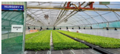
Nursery greenhouse irrigation system.jpg
