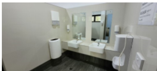
Handwash basins in bathrooms next to GLT Plant.jpg
