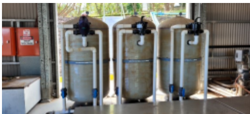
On-site water filtration system.jpg
