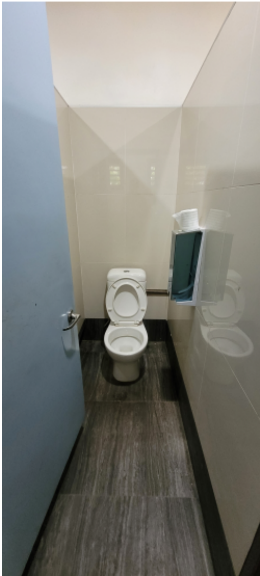
Toilet in bathrooms next to GLT Platn.jpg
