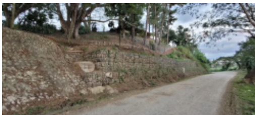
Stormwater drains leaving the site on eastern side.jpg
