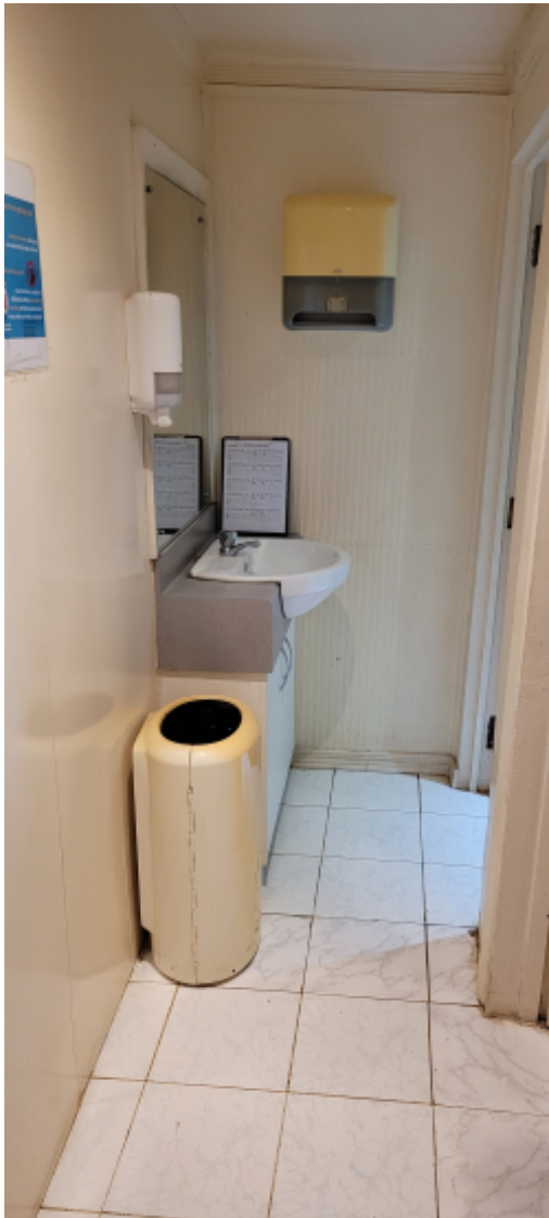
Handwash basin in bathroom near greenleaf tobacco drier.jpg
