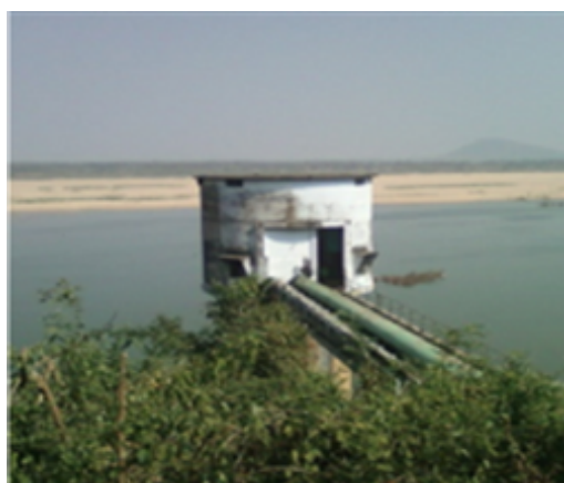
River water intake well at Iruvendi.png
