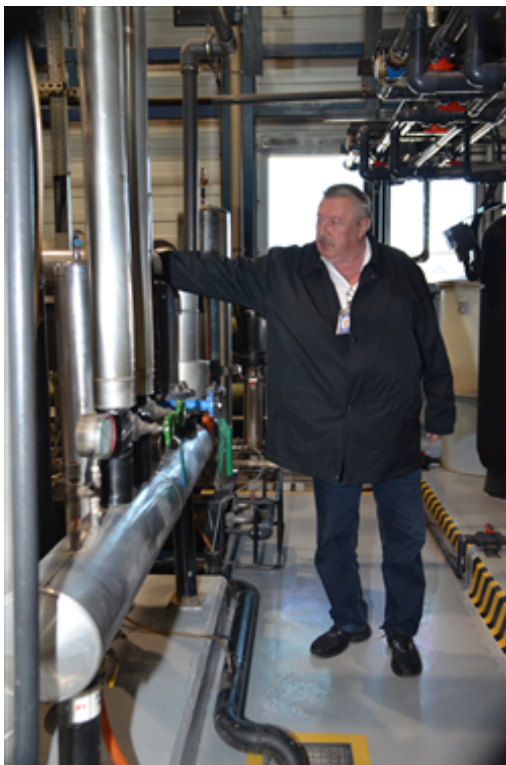
Boiler House - RO Water Distribution point.JPG
