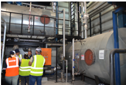
Boiler House - Condensate tank.JPG
