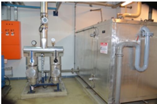
Heating point - Condensate Tank and Pumps.JPG
