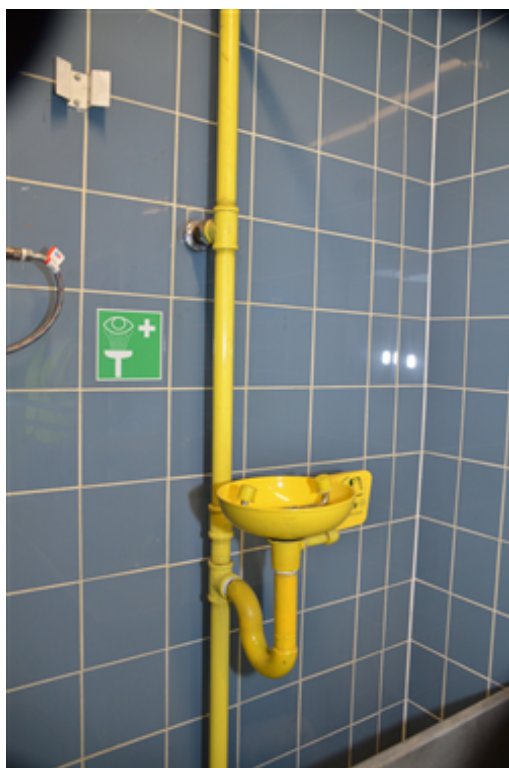
AC.PC warehouse - eye washing system.JPG
