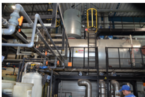
Boiler House - Feed water tank.JPG
