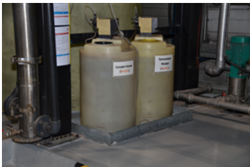
Boiler House - Chemical dosing pumps.JPG
