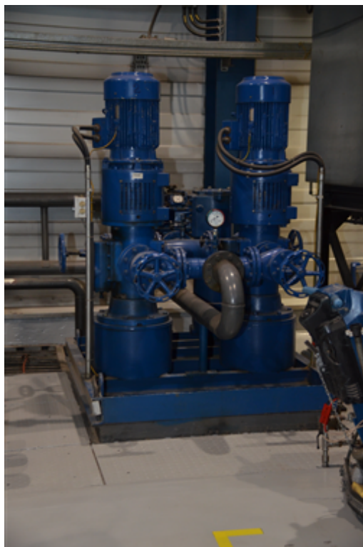
Boiler House - Diesel pump.JPG
