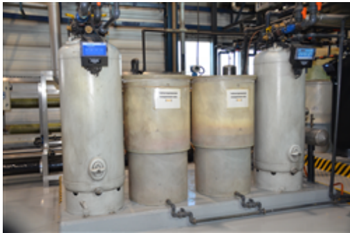
Boiler House - NaCl Tanks.JPG
