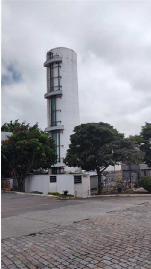
Water reservoir for general consumption and fire response.jpeg
