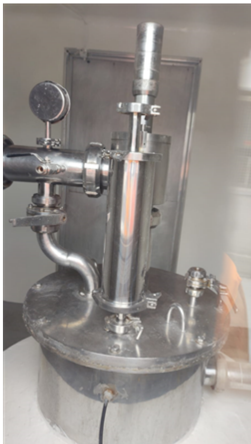
Yguaba well head with microbiological filter to filter the air.jpeg
