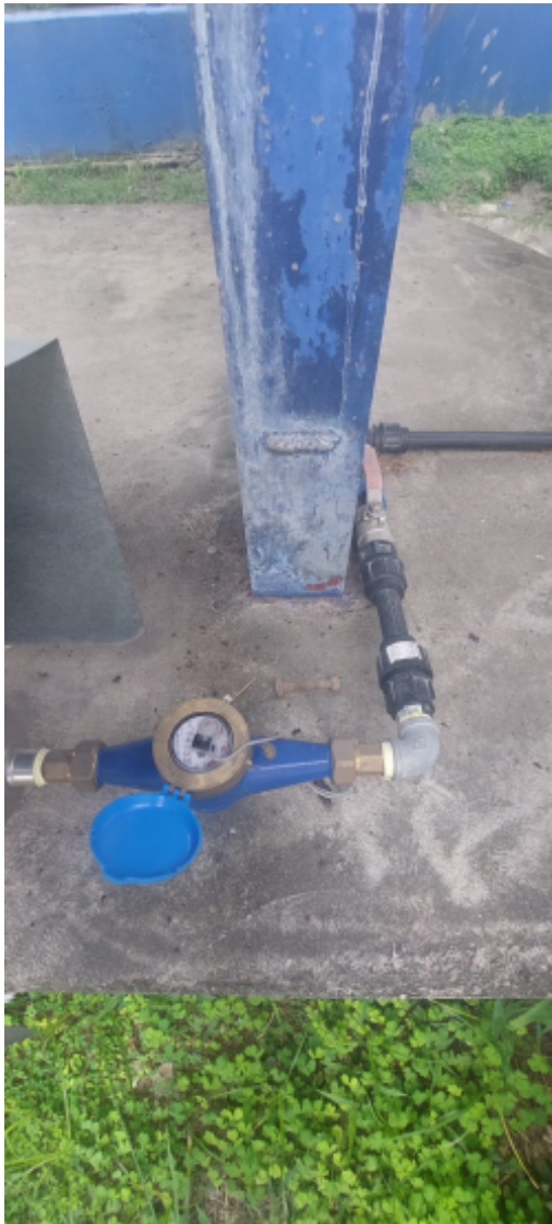
Water meter for rainwater.jpg
