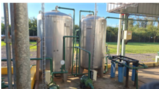
Sand, carbon and polypropylene filters.jpeg
