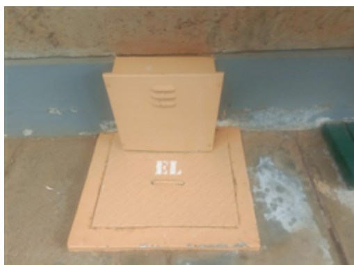
Electricity cable inspection manhole outside accounts block.jpg
