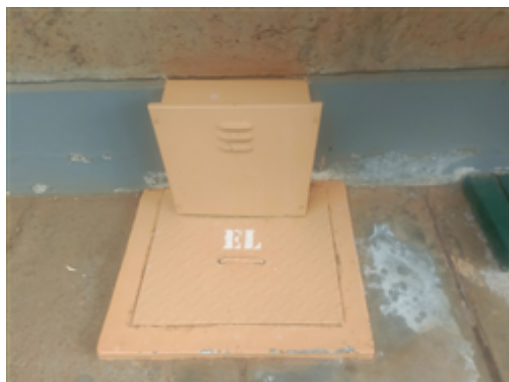
Electricity cable inspection manhole outside accounts block.jpg
