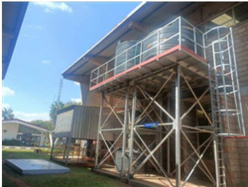
Gray water recycling sedimentation and collection tanks.jpg
