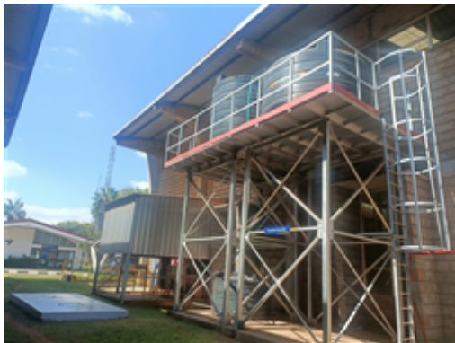
Gray water recycling sedimentation and collection tanks.jpeg
