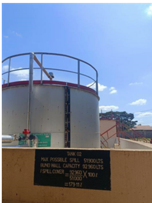
Tank 2 Bundwall containment.jpg
