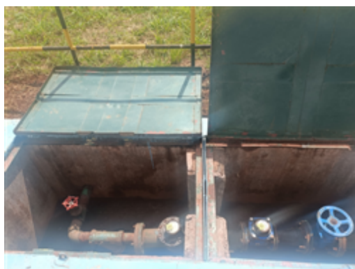
Municipal meters inlet into site.jpeg
