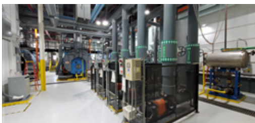
20240730_093222 High Temp Hot Water Pumps Boiler Plant.jpg
