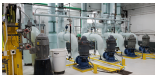
20240730_093343 Condensing Water Pumps Central Plant.jpg
