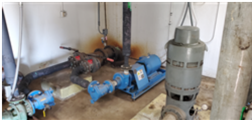
20240730_095740 Back-up Booster Pumps in Well House.jpg
