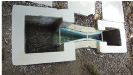
Flow metering of the treated effluent before its discharge Metering of the treated effluent.JPG
