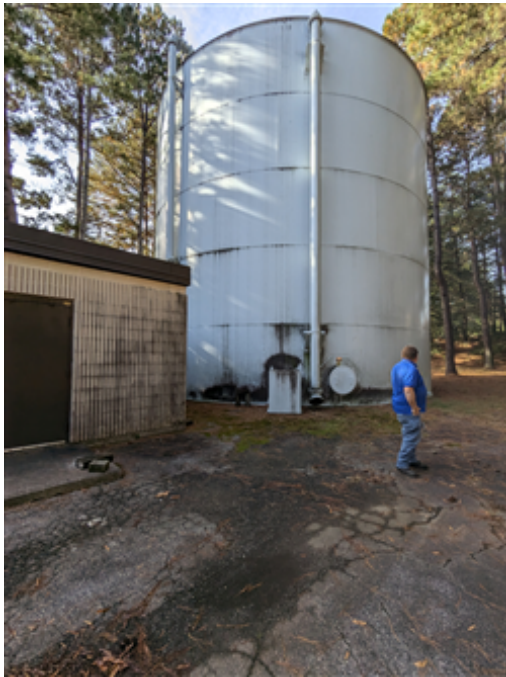
Fire suppression water tank.jpg
